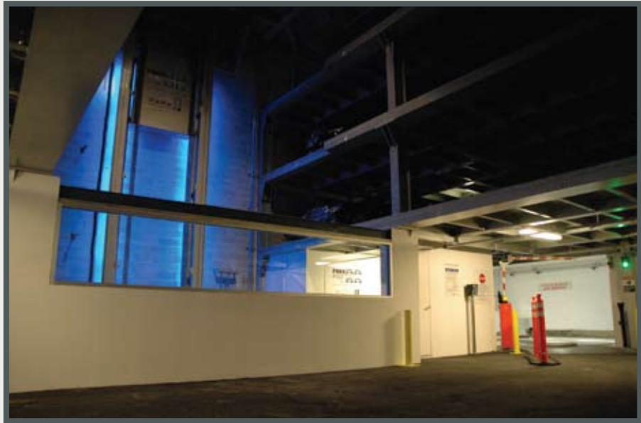
The One York residential condominium in New York City features a totally automated parking garage. Photo courtesy of Ryan Astrup, Park Plus, Inc.
